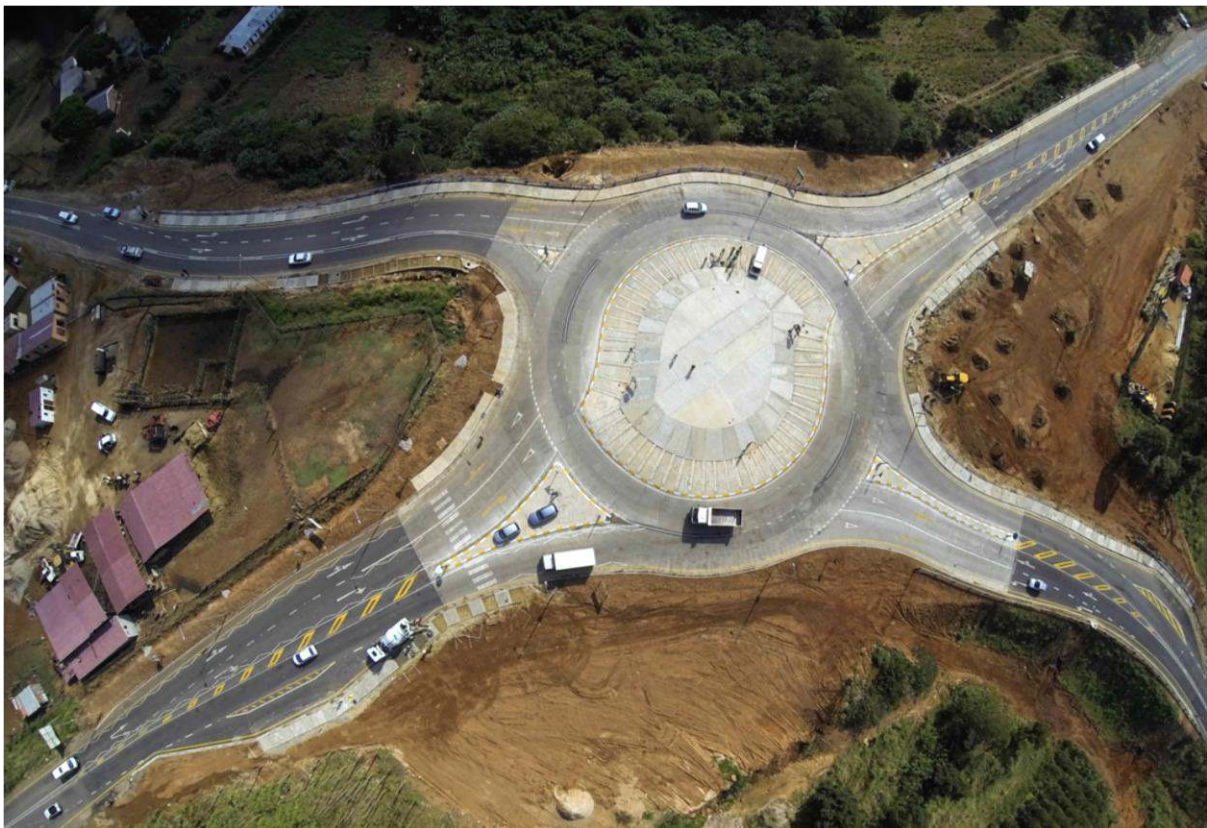
Figure 4-1: Completed R102 –Zululand University Turbo Roundabout
