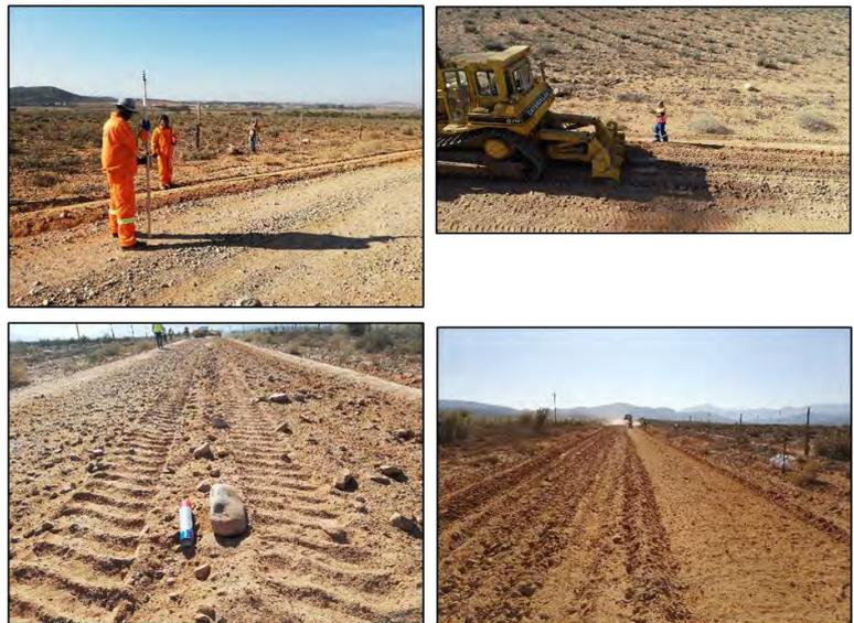
**Figure 7: Trial section construction sequence: Setting out (top left); Ripping the in-situ material (top right); Blading oversized material onto the roadbed (bottom left); Crushing of in-situ material (bottom right).**
