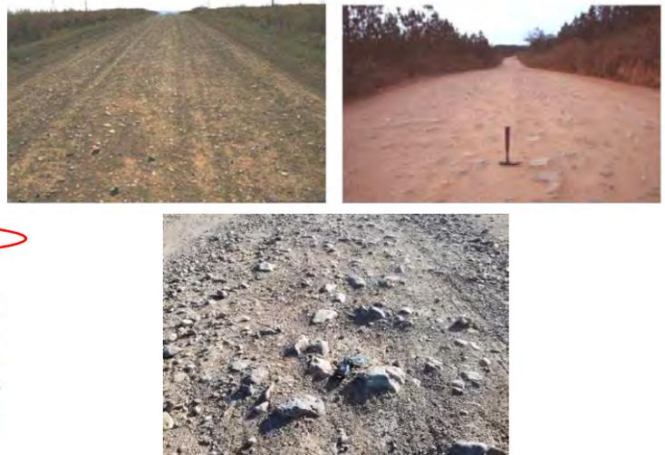
**Figure 2: Unpaved roads with stoniness fixed defects [3]**
